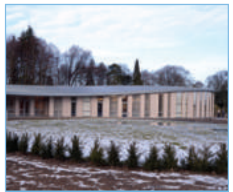
The new Linburn Centre
